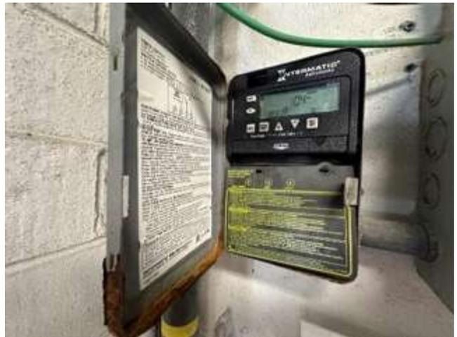
Photo 40 Corroded lighting controller
