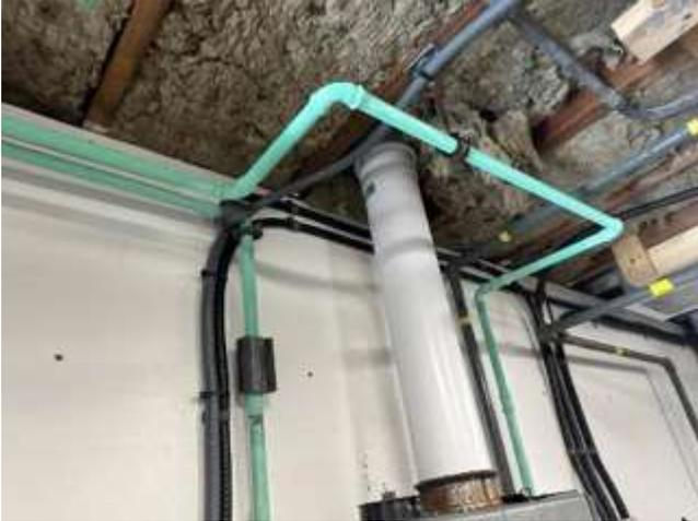
Photo 21 Domestic water copper piping
