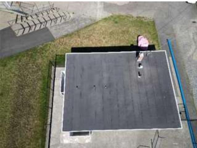
Photo 7 Modified bitumen roof
