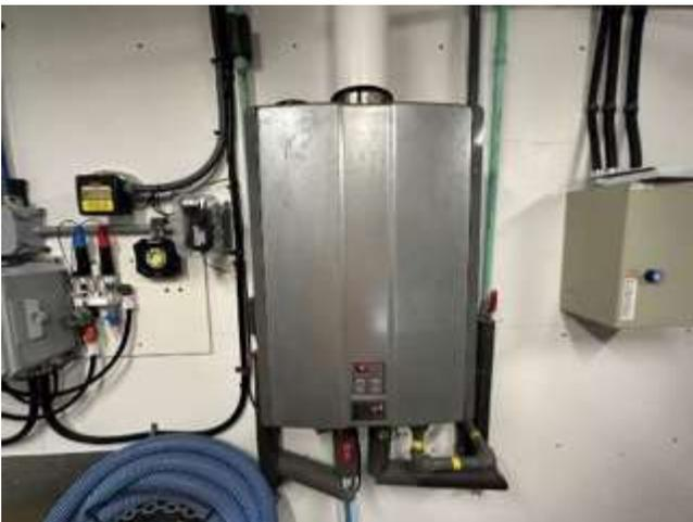
Photo 23 Gas-fired water heater
