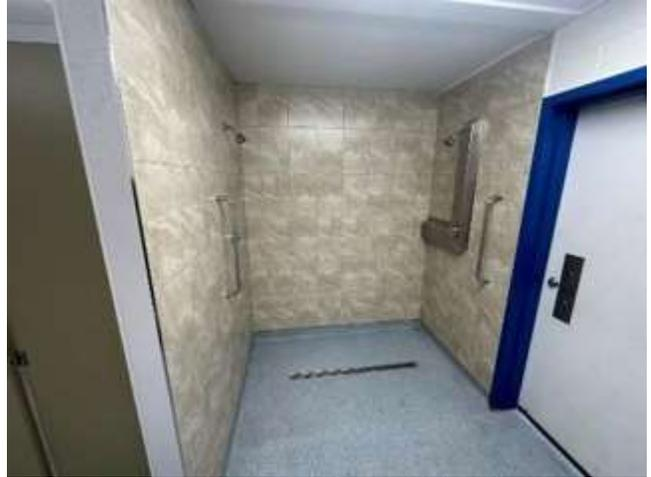
Photo 14 Shower stall with tile finish and epoxy flooring
