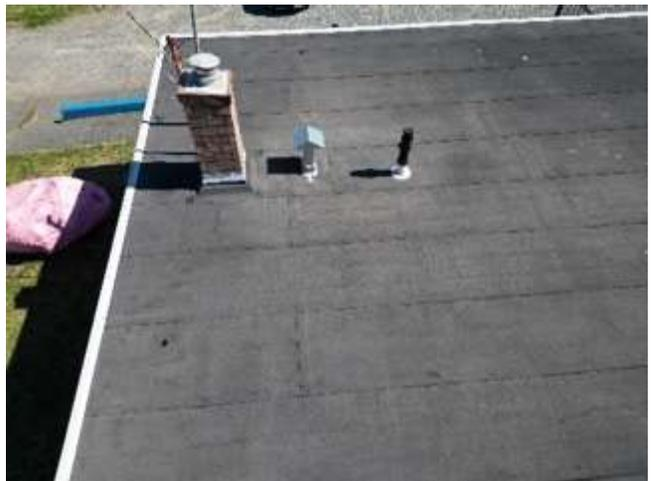
Photo 8 Exhaust, sanitary and roof vents
