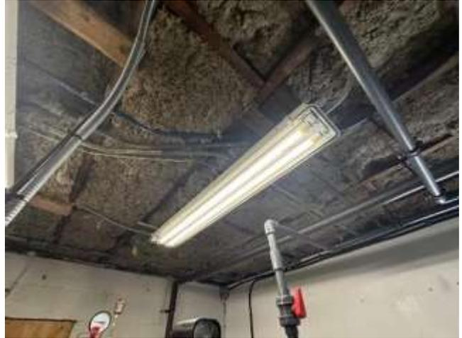
Photo 2 Wood joist roof deck
