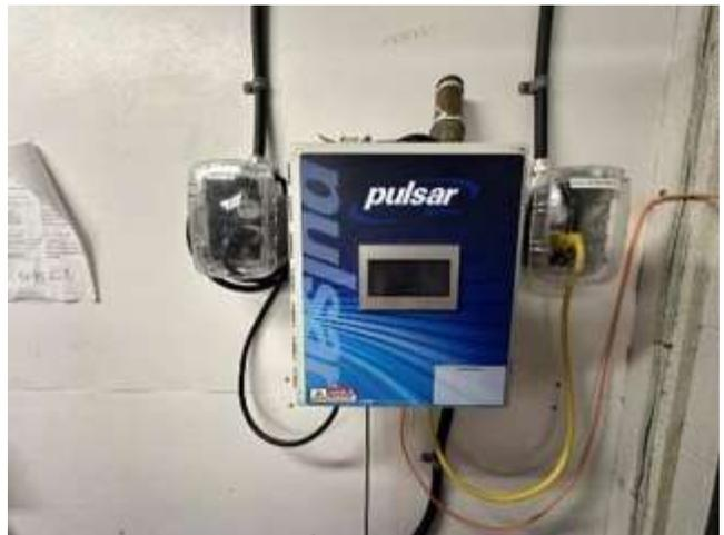
Photo 36 Chlorination system controller
