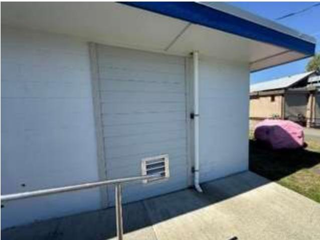
Photo 3 Fiber cement siding with louvre
