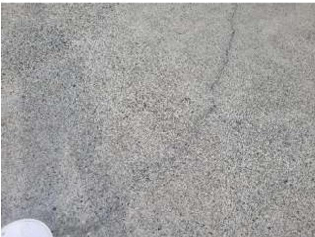
Photo 51 Pool walkway cracks
