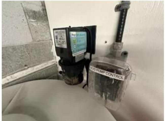
Photo 28 Acid pump controller
