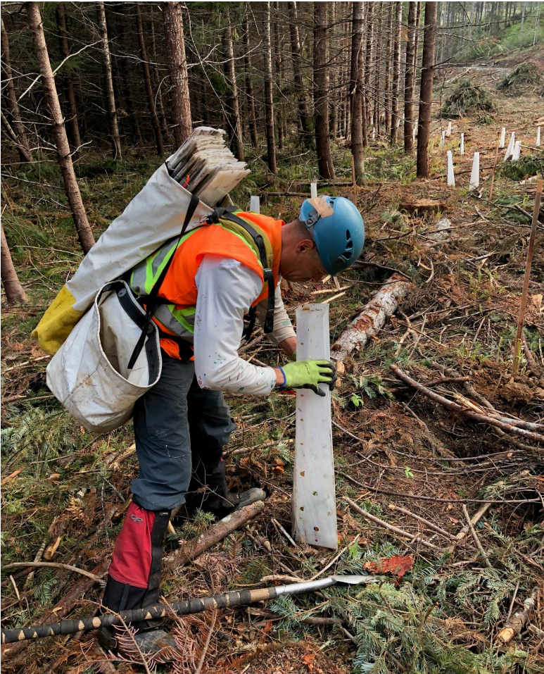
Tree Protector Installation – Maple Mountain – M-403
