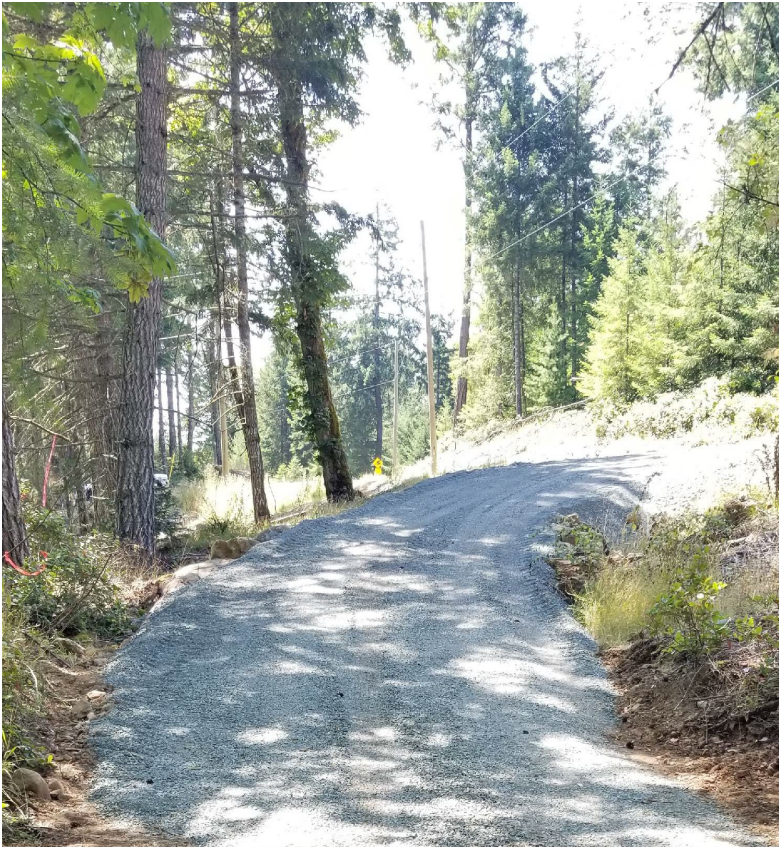
Fire Protection – Water Access Road Improvements – Stoney Hill
