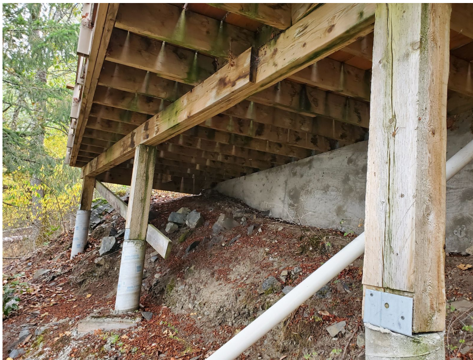
Figure 3 - Deck built on concrete piers
