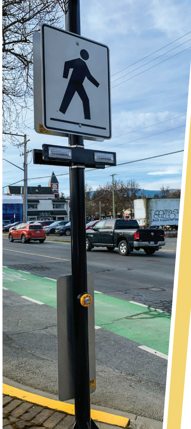
RECTANGULAR RAPID FLASHING BEACON (RRFB) RECENTLY INSTALLED ON CANADA AVENUE
