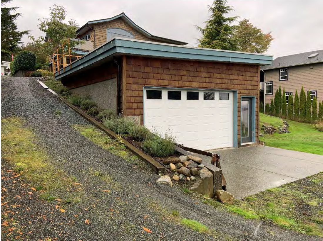
Photo 2.2.2: Existing garage and driveway, looking northwest.
