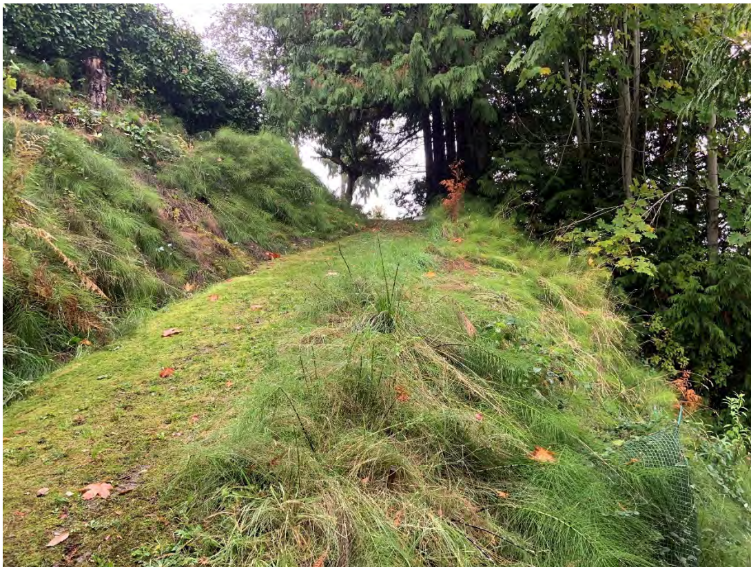
Photo 2.2.4: Slope conditions and trail, looking north.
