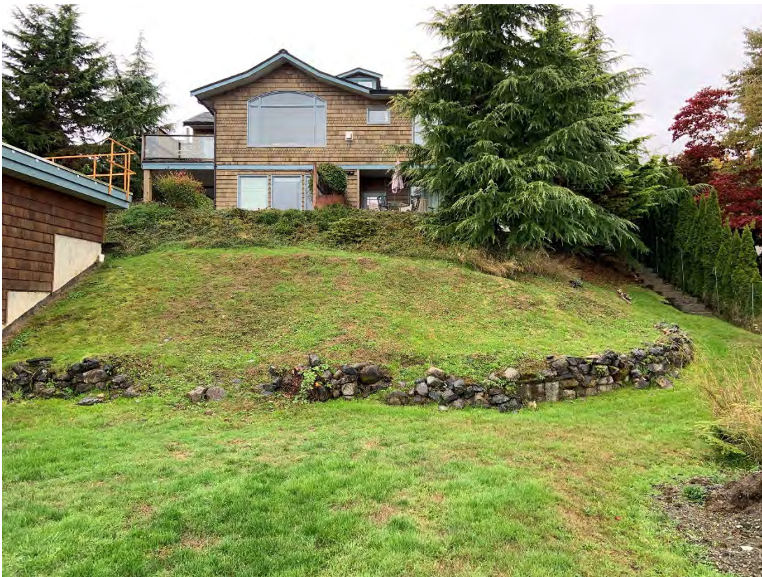
Photo 2.2.1: Existing residence as viewed from the proposed building area, looking west.
