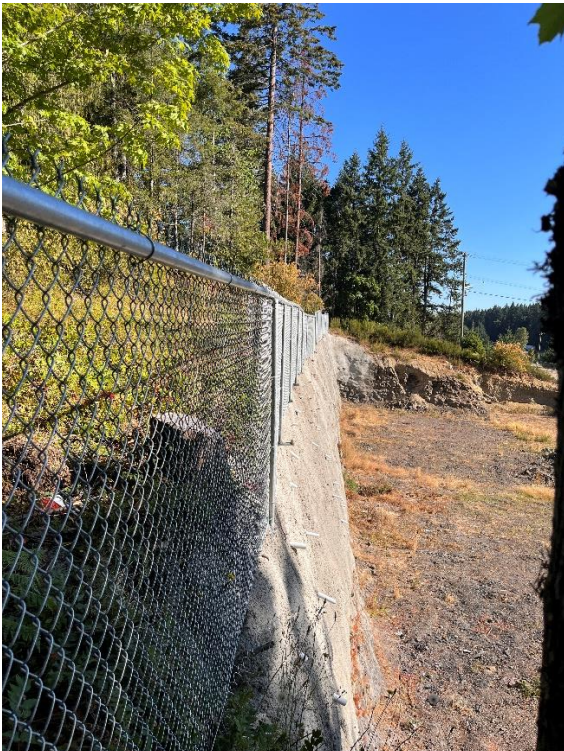
Photo 2 - Installed chain link fence, August 2023
