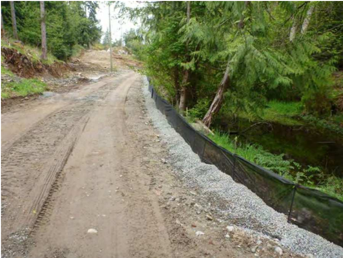
Figure 4. Two examples of silt fences installed with filtering pea gravel berms
