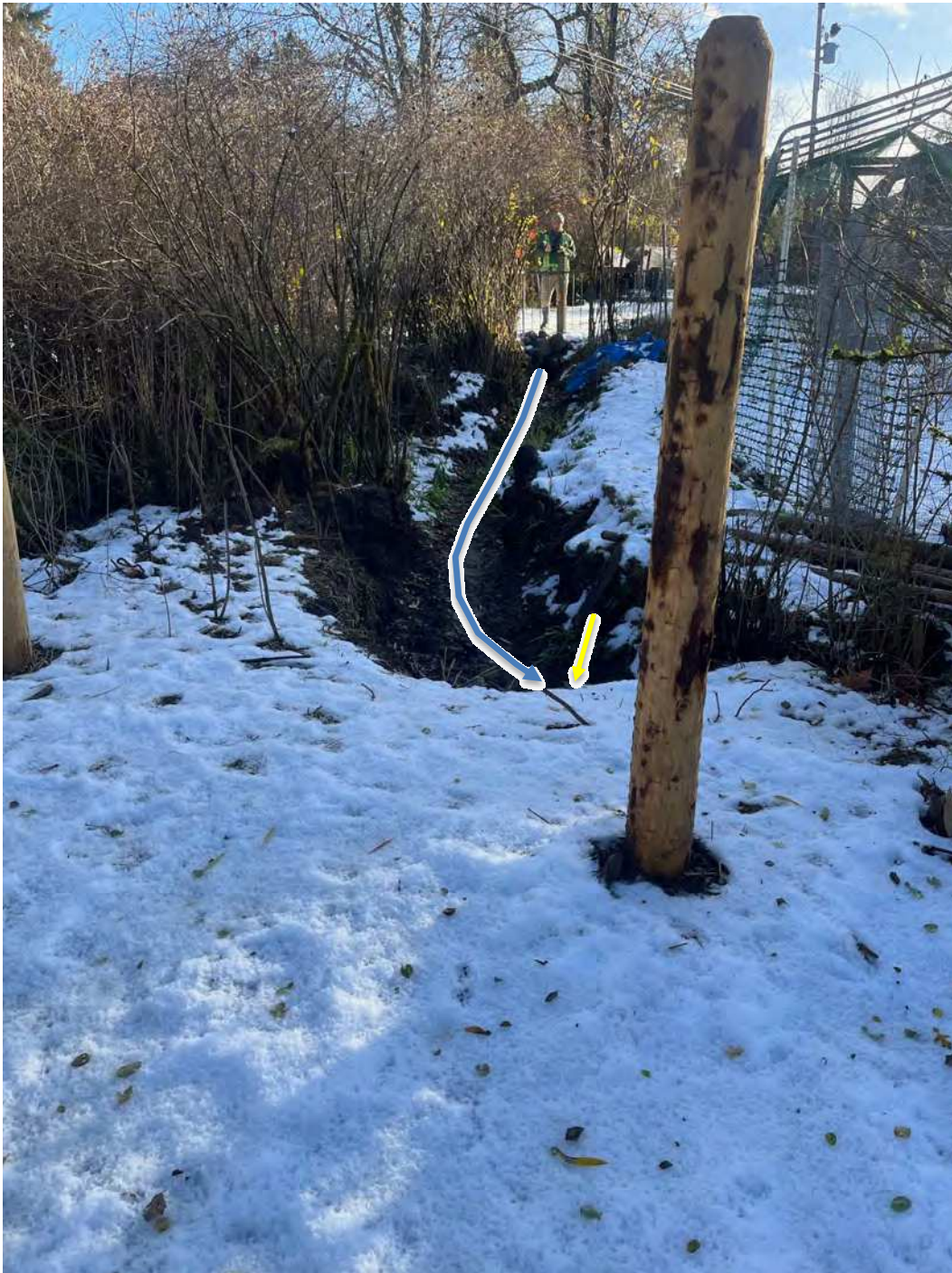
Figure 13. Looking upstream (southeast) at the recently daylighted stream channel on 1937 Maple Bay Road (Figure 10). Yellow arrow indicates the buried culvert inlet.
