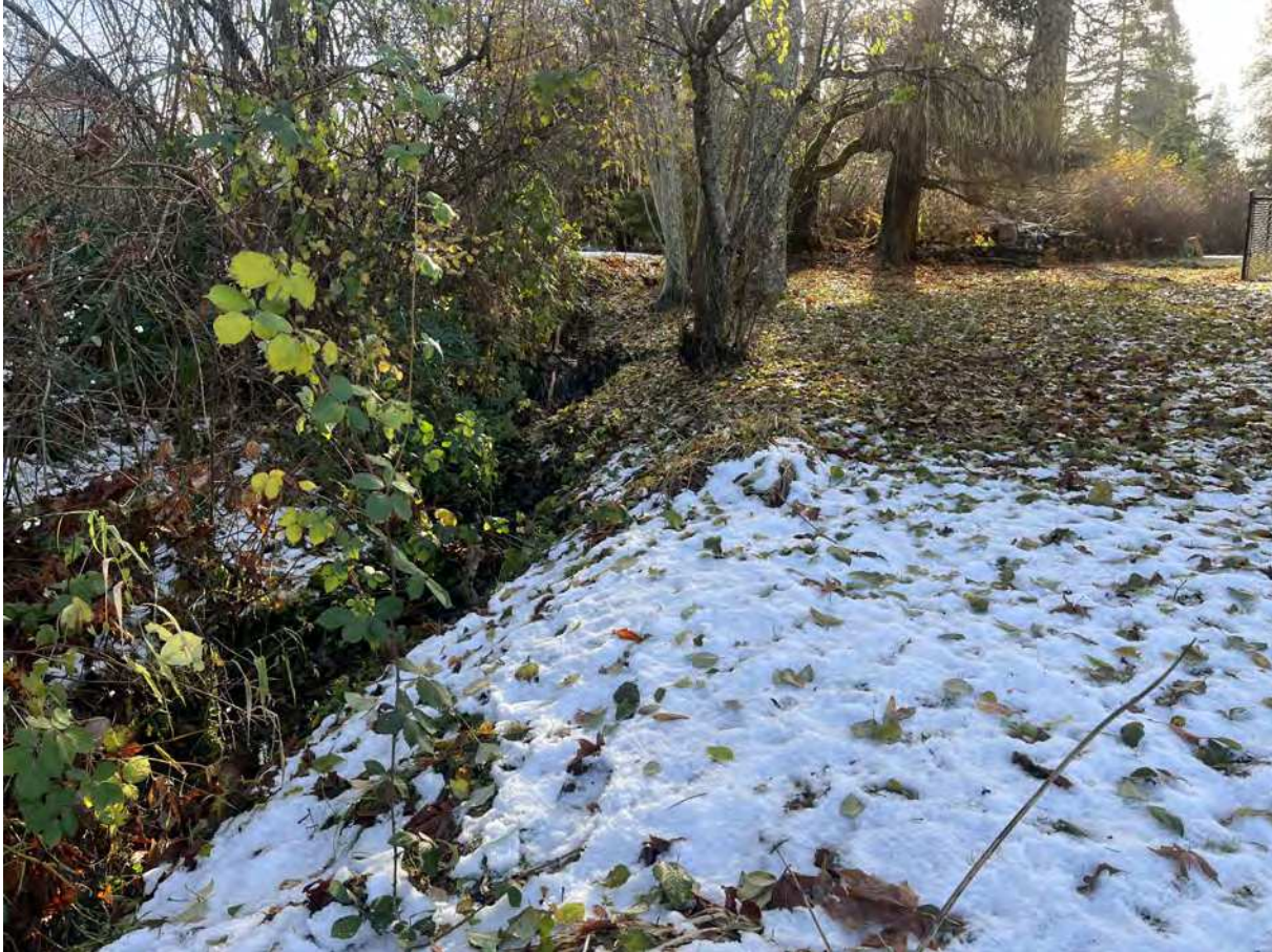
Figure 16. Looking upstream (south) at the moderately entrenched Ditch 1 on 1949 Maple Bay Road. Note the turf lawn and copse of trees on the west side of the channel. The culvert discharge shown in Figure 15 lies to the left of this image.
