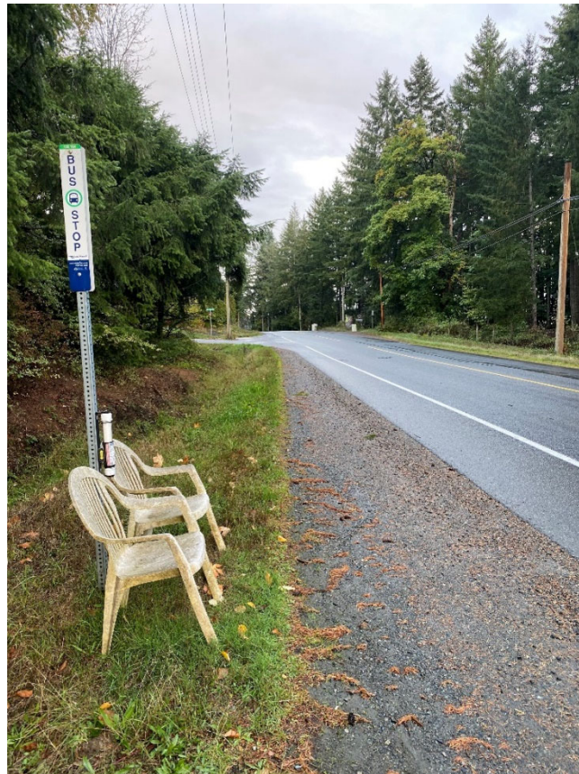
Example of Existing Bus Stop Infrastructure at North Cowichan Stops
