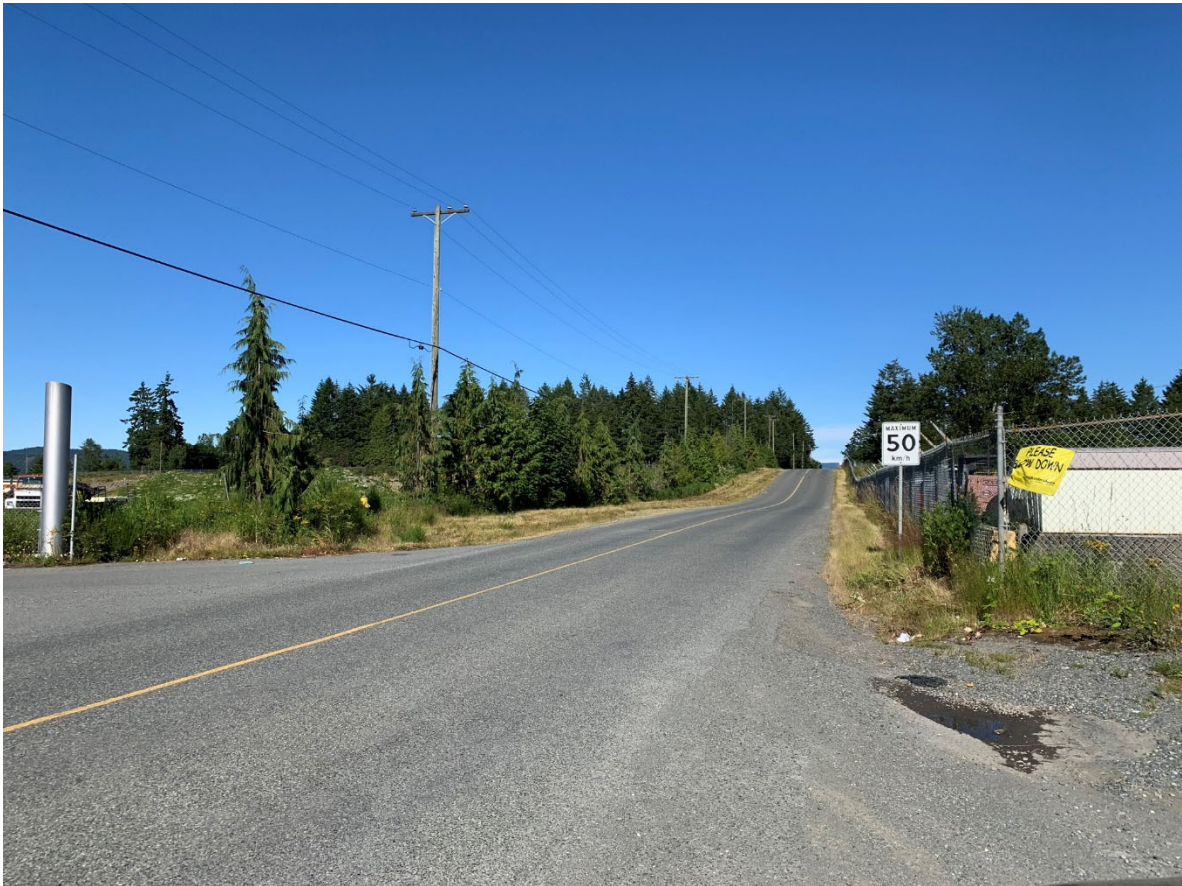
Drinkwater Road near Highway 18, where no pedestrian facilities are currently available
