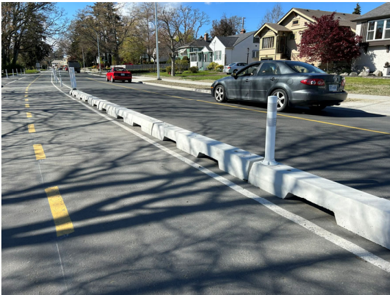
Examples of quick builds using concrete curbs (left) and plastic delineators (right)
