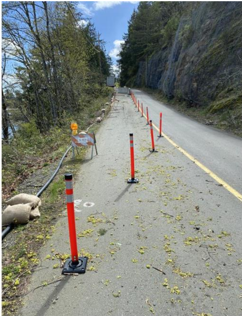
Figure 2 – Genoa Bay Road looking north (right) and south (left) through an unstable road section with the water main temporarily relocated on top of the road (steep slope next to the water main).
