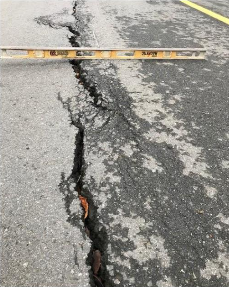
Figure 3 – Large settlement cracks looking south through an unstable road section (steep slope to the left).
