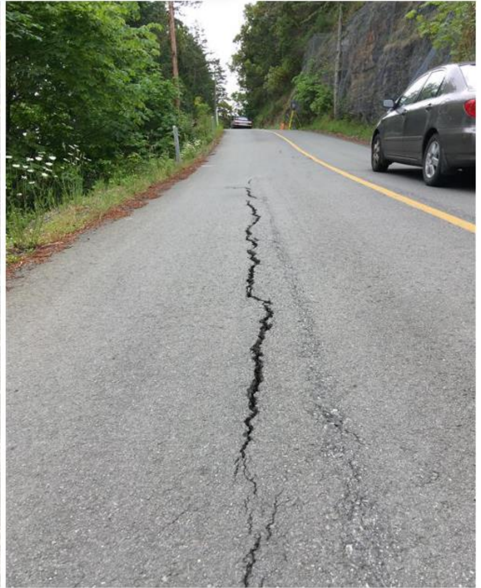
Figure 3 – Large settlement cracks looking south through an unstable road section (steep slope to the left).
