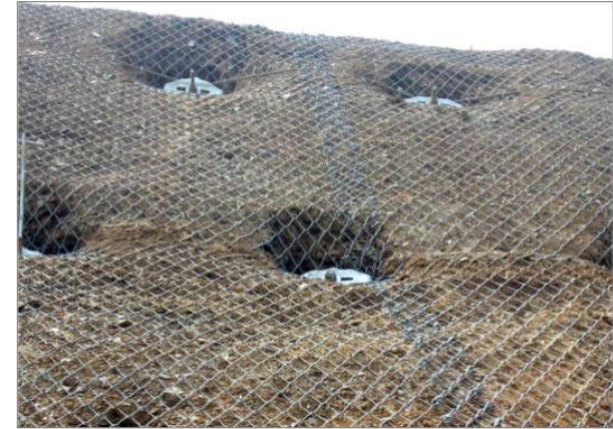
TECCO® system correctly installed and pretensioned
