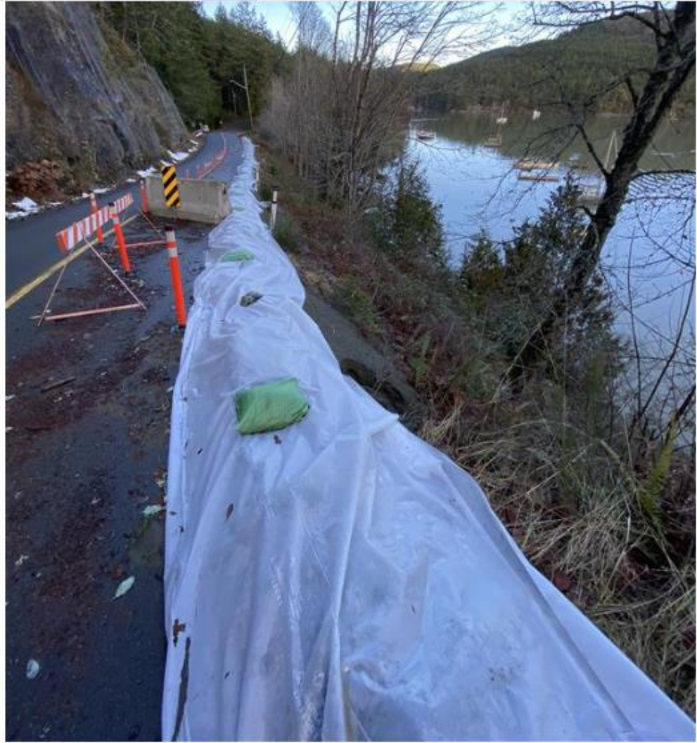
Figure 2 – Genoa Bay Road looking north (right) and south (left) through an unstable road section with the water main temporarily relocated on top of the road (steep slope next to the water main).
