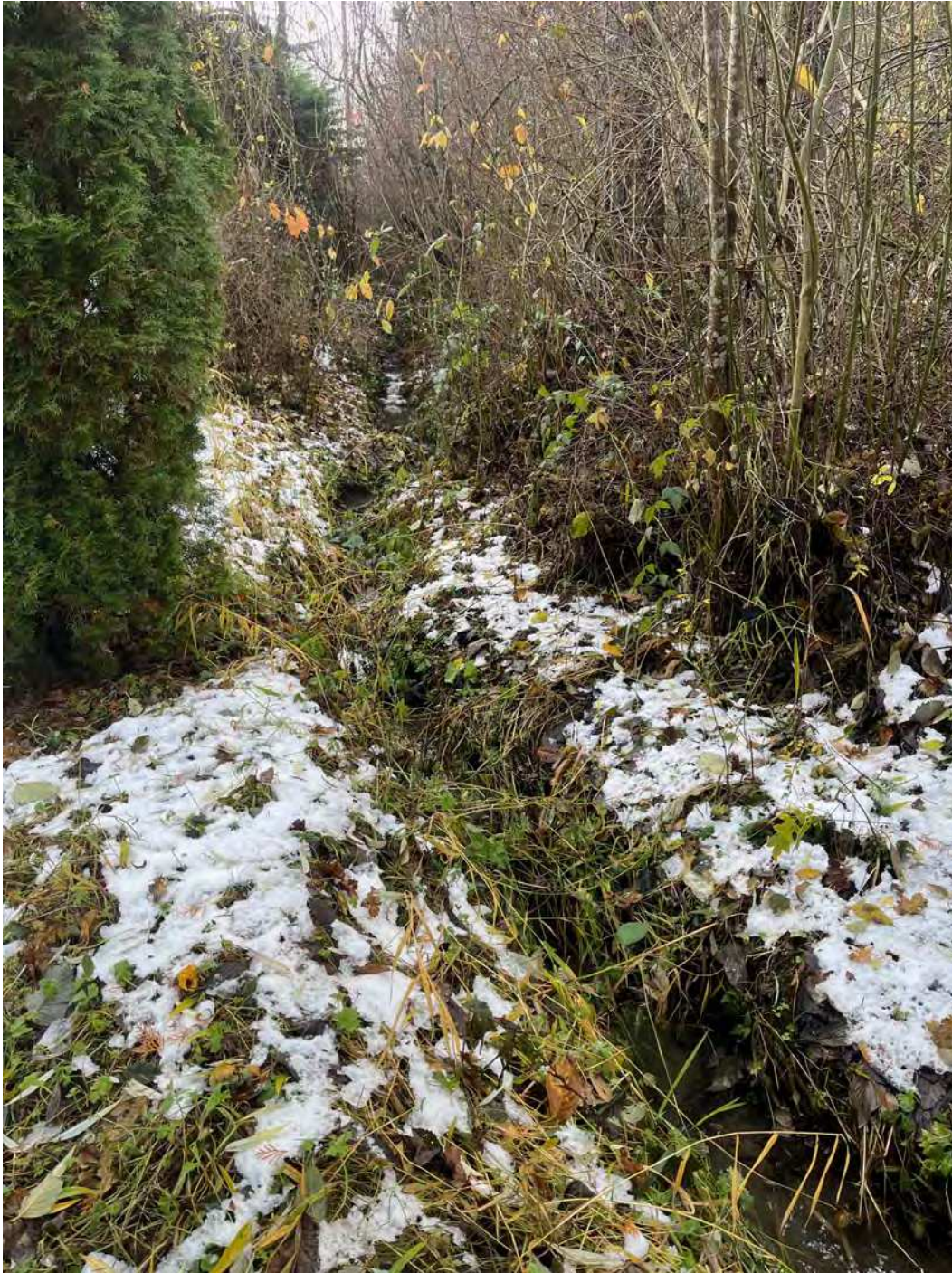
Figure 23. The uppermost section of Ditch 1 (~50m downstream of the culvert outlet under Maple Bay Rd) has a non-native cedar hedge on the east bank and a shrub-dominated vegetated west bank. The channel remains entrenched, with agronomic grasses assisting in providing some bank soil stability. This section has considerably more shading of the channel than the reaches downslope. There is moderate blackberry invading the hedge and shrub community.
