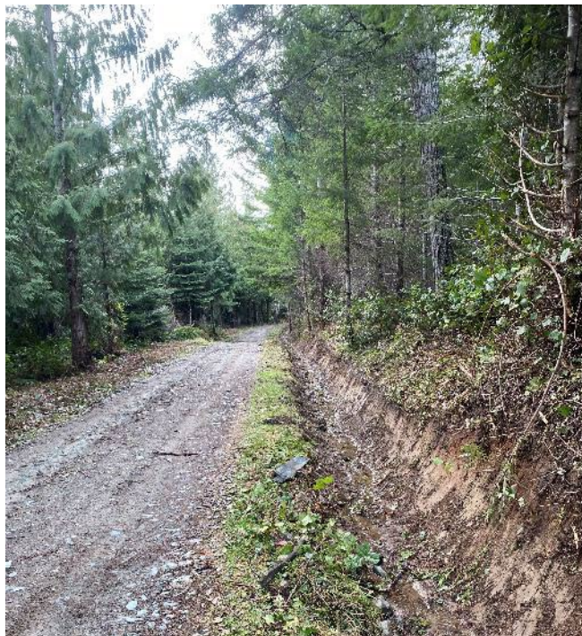
Ditch Cleaning – Mount Richards
