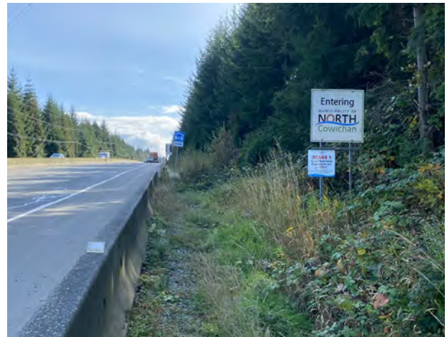
Existing gateway sign marker at the Highway 1 North Gateway into North Cowichan.
