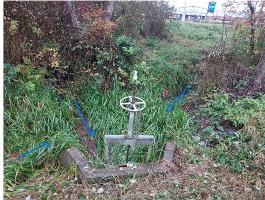
Figure 31: On a regular basis, site BWQ1US water flows directly from the Beverly Street culvert and adjacent Beverly street ditch (flows east toward round about), through this dike culvert, and does not flow through the wetland
