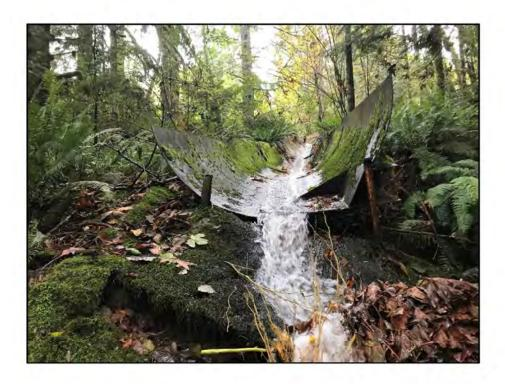
Photo 4. The metal spillway where the tributary stream flows over the top of the steep slope that leads down to the Chemainus River to the southwest of the parcel.
