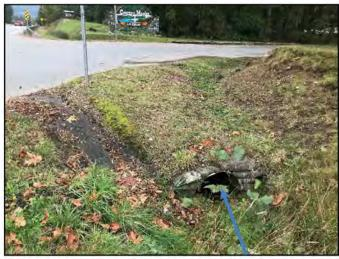
Photo 28. Showing the culvert crossing the entrance road from the highway into Country Maple RV Resort.
