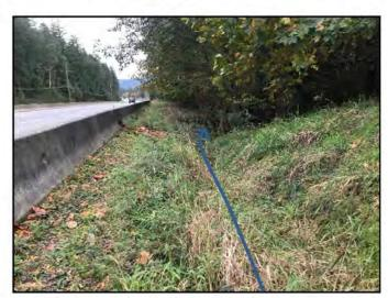
Photo 30. The highway ditch terminates by fanning out over the top of the slope leading down to the property just south of the subject parcel. No channel present over the slope.
