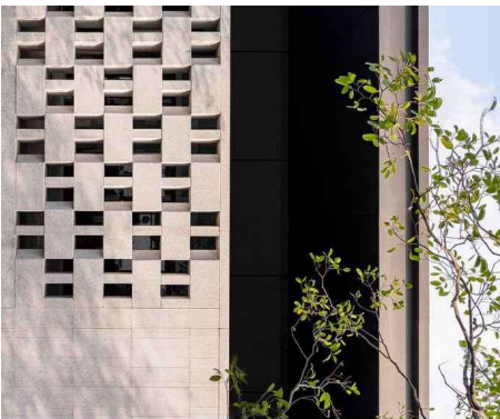
BREEZE BLOCK WALL
