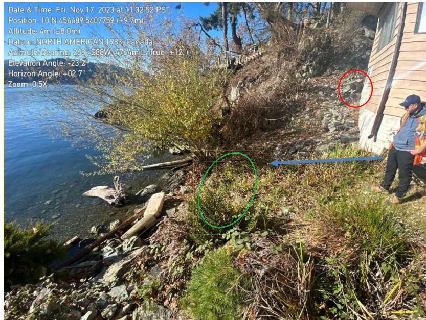
Photo 17. West-facing view of backshore area. November 17 th , 2023. See culvert outlet (circled in red), drainage pathway that surfaces beneath house (shown in blue) and gutter drainage all collecting in one area compiled with groundwater seepage that is causing slope creep in the area circled in green. A seawall ~3 m long comprised of boulders with geotextile and drain rock in behind is proposed to stabilize the area from future erosion.
