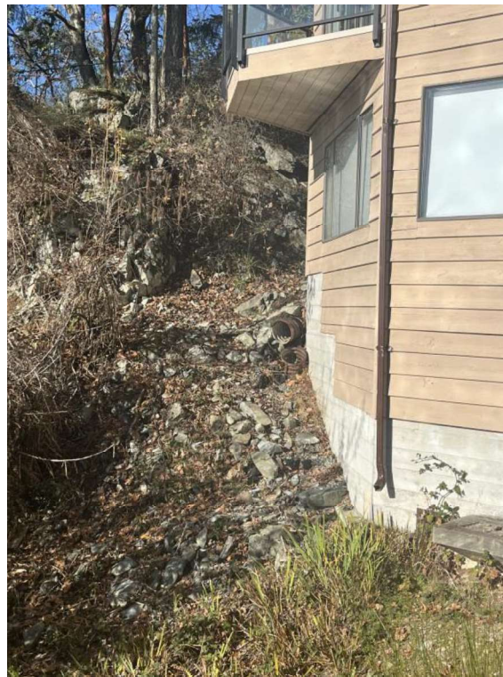
Photo 13. Drainage/culvert alongside west side of house from driveway. November 17 th , 2023.
