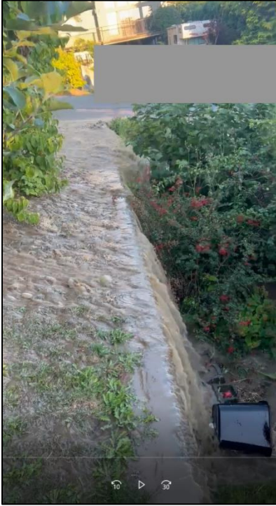
Figure 4 – Flooding downstream of water main break over retaining wall.
