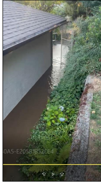
Figure 5 – Flooding downstream of water main break over retaining wall and into backyard.
