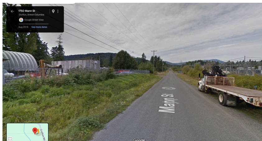
Figure 6: Proposed tower location on the left, facing west on Main Street towards the Substation on the right.
