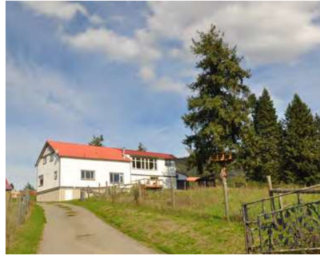
Figure 3.18: Existing rural residence.
