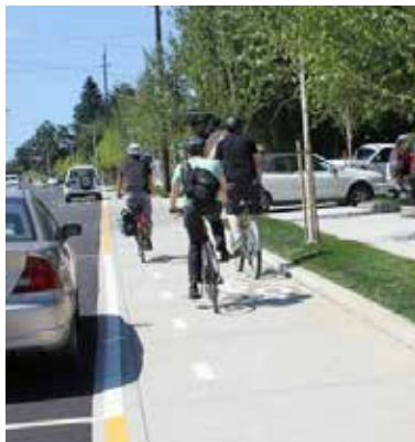
A raised separated bicycle facility
