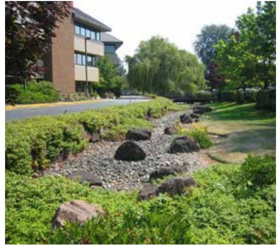
A landscape-based stormwater detention area
