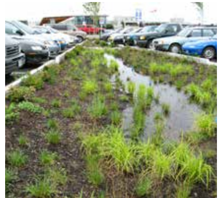
An on-site raingarden receiving parking lot run-off
