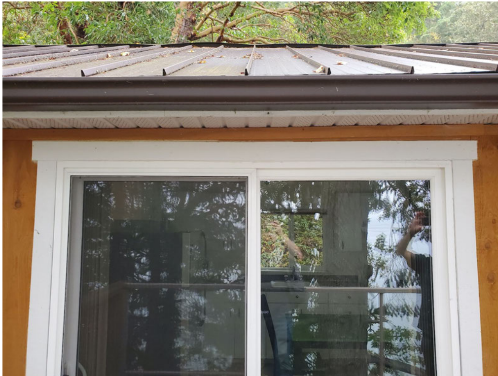
Figure 4 - Sliding door trim angled in relation to the roof
