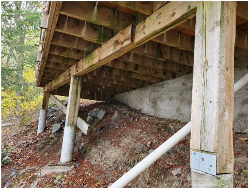
Figure 3 - Deck built on concrete piers
