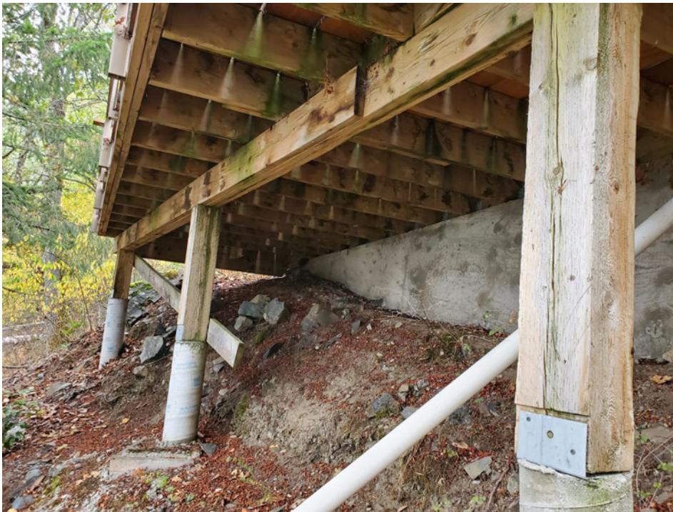
Figure 3 - Deck built on concrete piers
