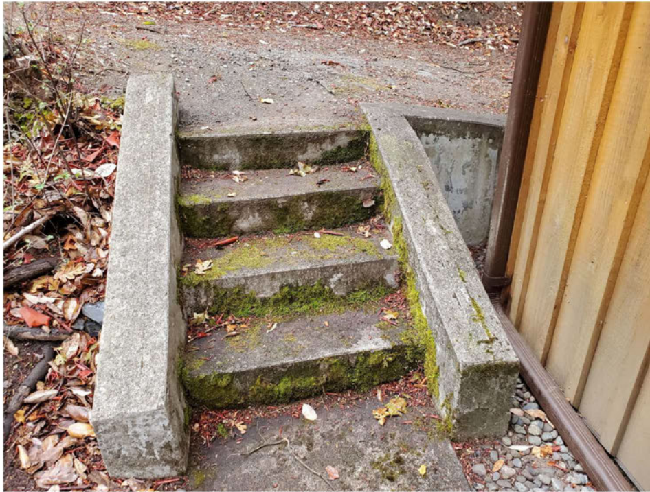
Figure 2 - Exterior concrete stairs
